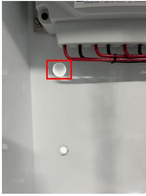
To remove the knockout plugs, use a screwdriver and mallet to strike the BOTTOM of the plugs. Avoid striking the knockout plugs at the top, as they are attached to the enclosure at the top.
